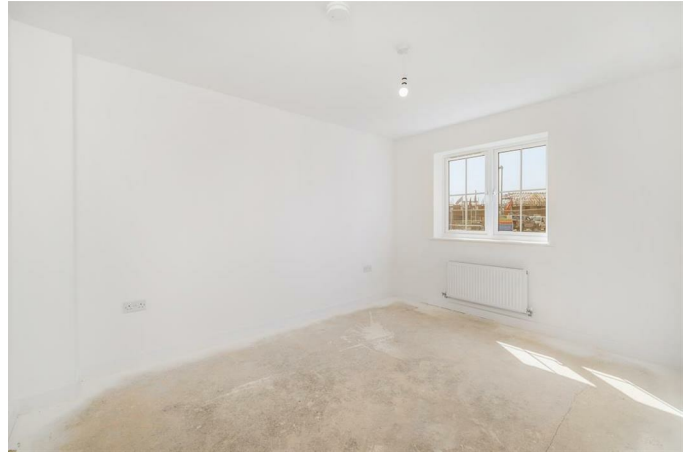
UPVC window to front. Radiator.
